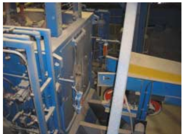
P12" unit at curve-sawing VSA outfeed
